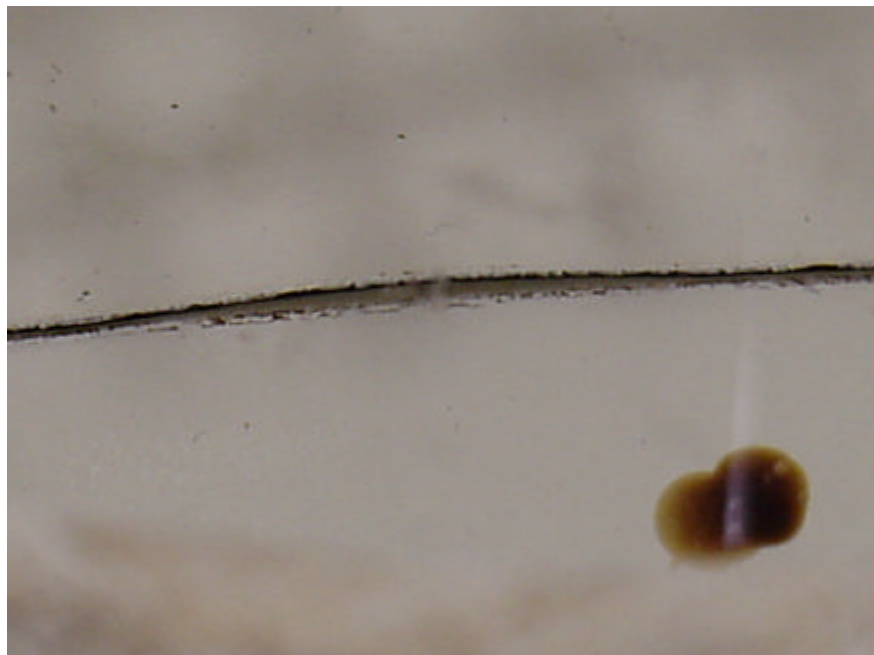
Figure 6. The lap joint in Cell D coated with 610 tape, showing partial joint separation.
